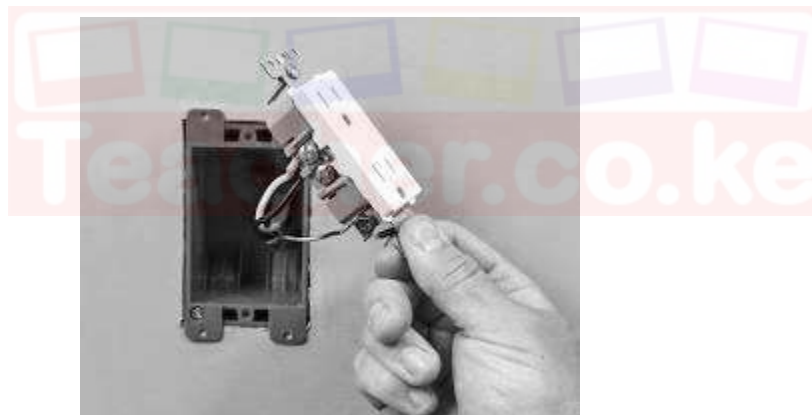
Installed wall socket
