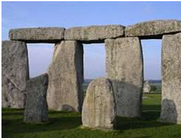
Fig. 1.5: Stonehenge, an example of Neolithic architecture post and lintel construction
